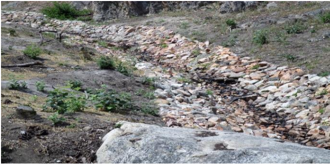
Inlet works Wittewater and rock paved canal
