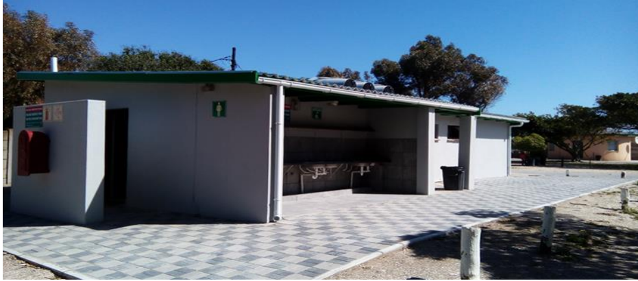
Upgraded ablution facility at DKB
