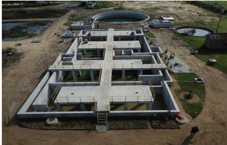
Upgrading of Porterville Sewerage Works
