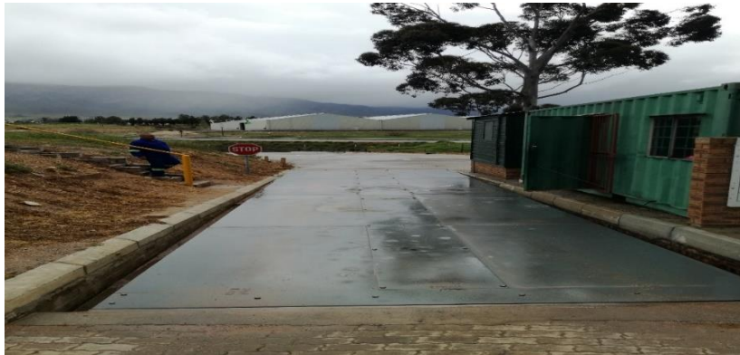
Photo of weighbridge
