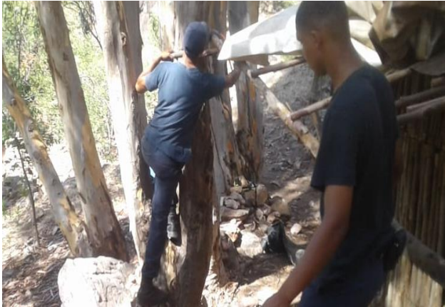
Law Enforcement busy with the removal of illegal structures
