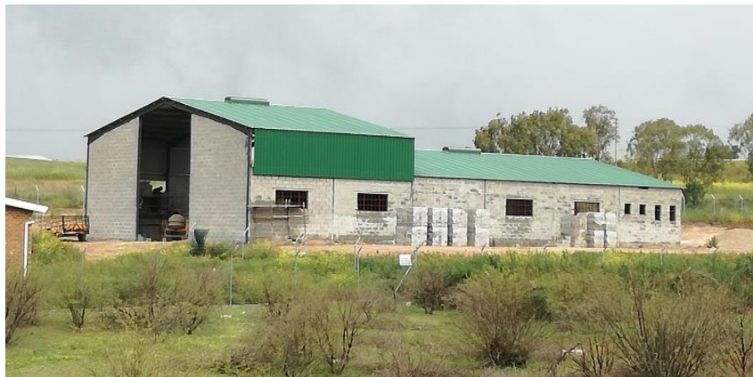
Photo of recycling plant under construction: Piketberg
