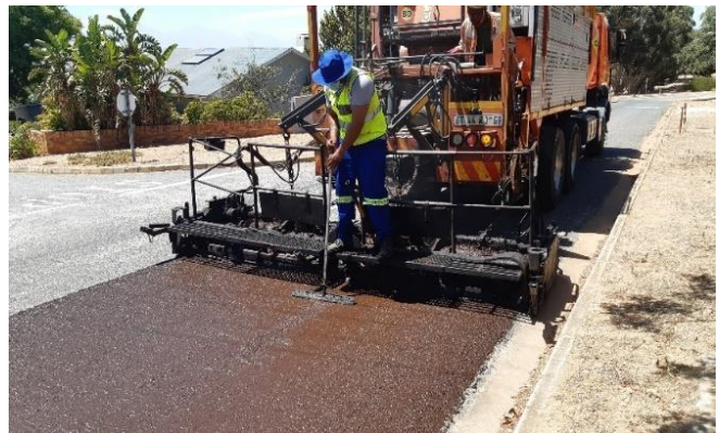
Road being ressealed in Piketberg as part of preventative maintenance
