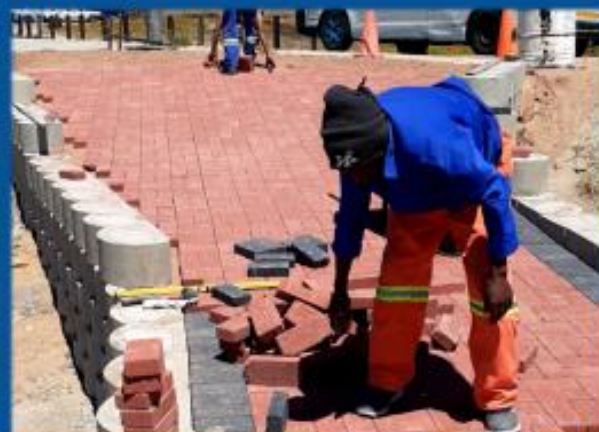
The Walkway RSEP project in Velddrif was completed in March 2021
