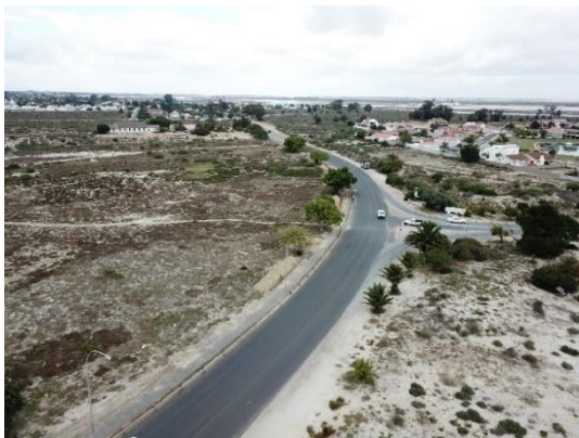
Section of Voortrekker Street in Velddrif ressealed
