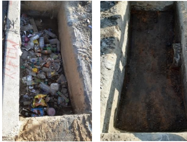
Storm water catch pit in Ward 4 before and after being cleaned
