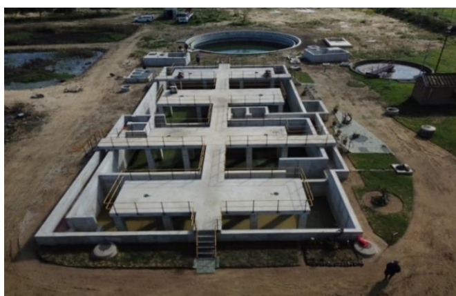
Upgrading of Porterville Sewerage Works
