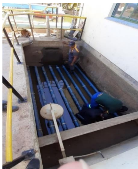
Piketberg WTW filter media being replaced
