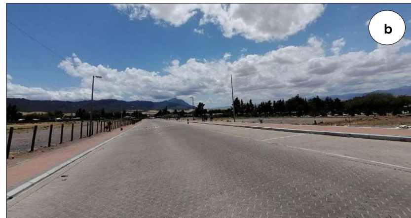
Plate 5a-b: Key public spaces such as the outdoor gym (a) and Calendula Street (b) have no tree planting, meaning that users are exposed to the harsh summer sun
