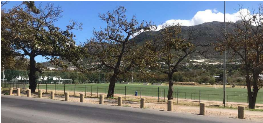
Image 8: Permeable fencing surrounding the Hout Bay sports precinct in Cape Town
