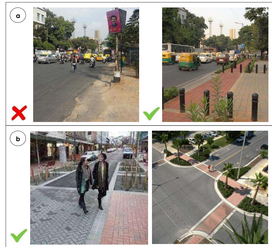
Figure 44: Specific guidelines for hard landscaping – use different materials, texture and colour to differentiate between hard surface functions (a); and use paving as a traffic calming measure (b)
