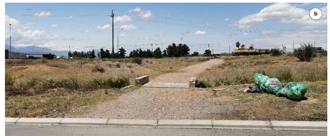
Image 27: The vacant land between the N7 and the cricket oval is sterile and presents a poor visual interface (a); the pedestrian pathway between Steynville and the N7 crossing (b)
