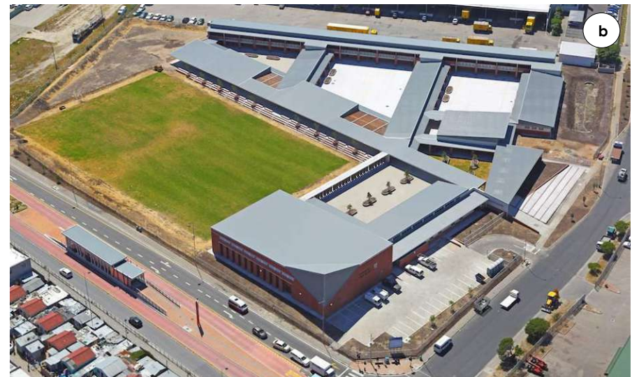
Image 26: Sinenjongo High School was designed so that it positively contributes to the public realm (a); the internal design is arranged around a hierarchy of sheltered courtyards (b)
