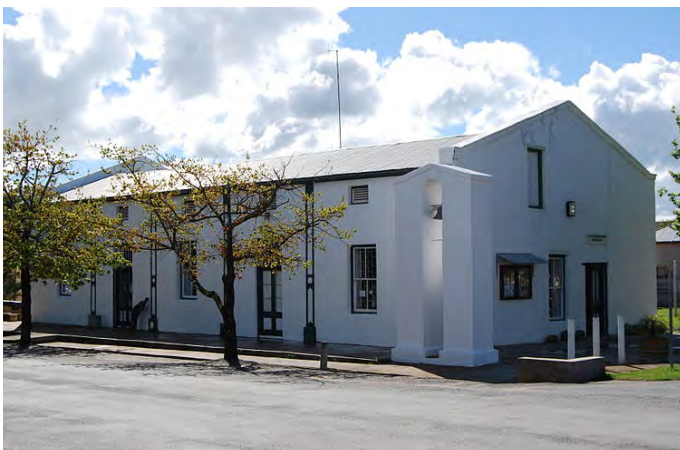
Photo 27. H1 - Mark Street - Former Police Station
