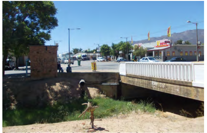
Photo 67. Voortrekker Street Bridge - Open Space Disconnected from CBD
