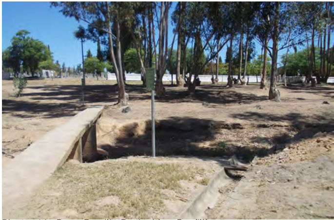
Photo 66. Poor Quality Pedestrian Facilities
