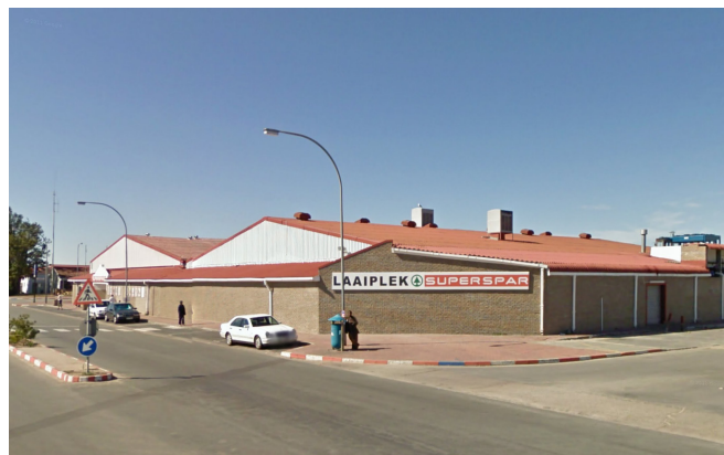
FIGURE 36. A BLANK BUILDING FACADE OF A RETAIL CENTRE IN LAAIPEK
