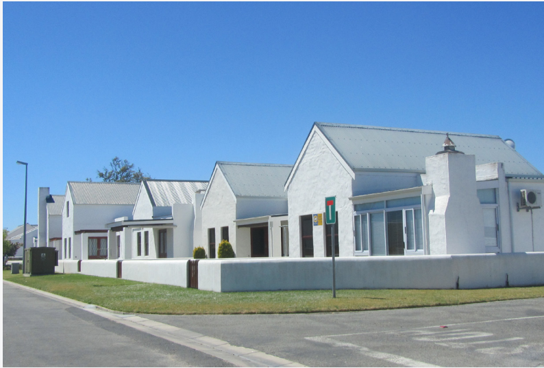
FIGURE 88. EXAMPLES OF THE UNIQUE BUILDING STYLE THAT IS ALREADY PROMINENT IN THE PRECINCT - USE OF LOW WALLS TO DEFINE THE ERF AND LOCAL MATERIALS TO STAY TRUE TO THE WEST COAST FEEL
