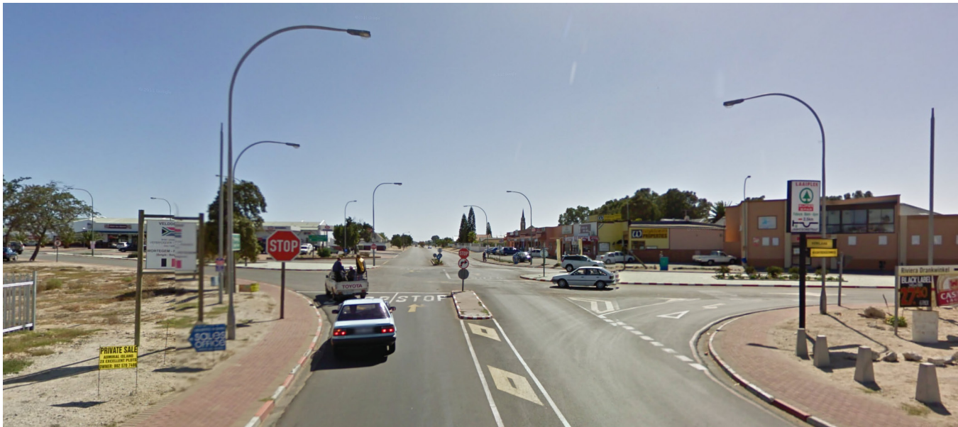
FIGURE 45. THE R27 - R399 INTERSECTION AT THE ENTRANCE INTO VELDDRIF
