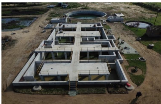
Upgrading of Porterville Sewerage Works
