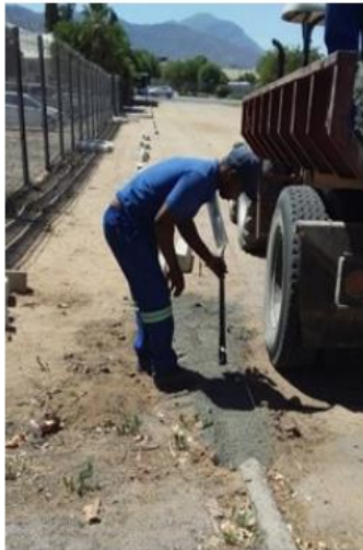
New road construction
