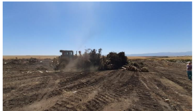
Photo of landfill site being cleared
