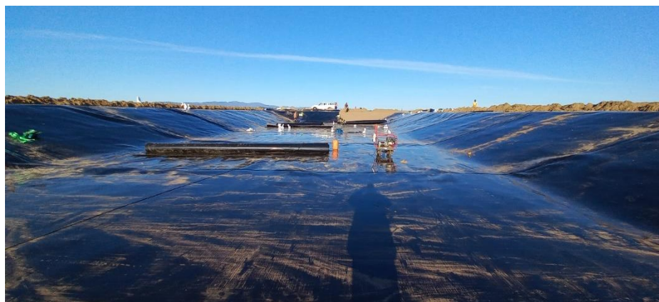
Upgrading of Dwarskersbos Sewerage Works
