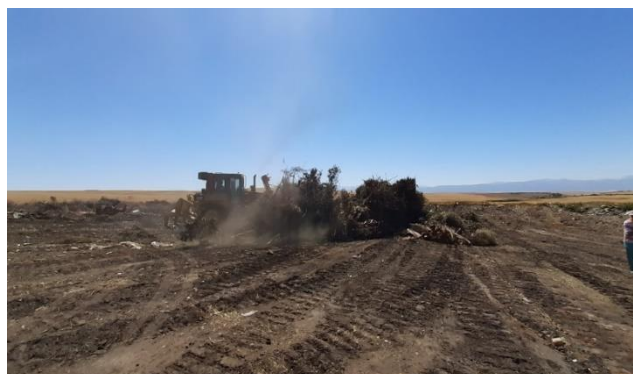
Photo of landfill site being cleared.
