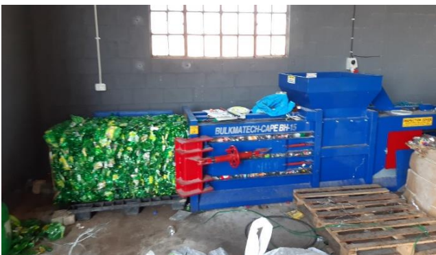
Photo of baler operating in the finished recycling plant
