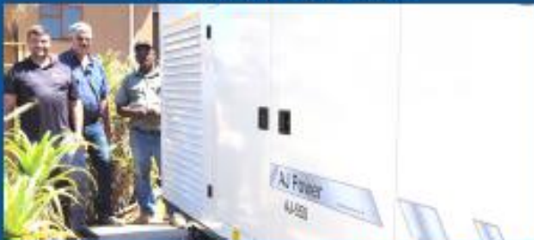
Bergrivier Municipality was awarded R3,4 million from the Western Cape Government which was used towards purchasing two large generators (550kWh and 330kWh) to ensure sufficient water purification for Piketberg.
