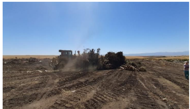
Photo of landfill site being cleared.
