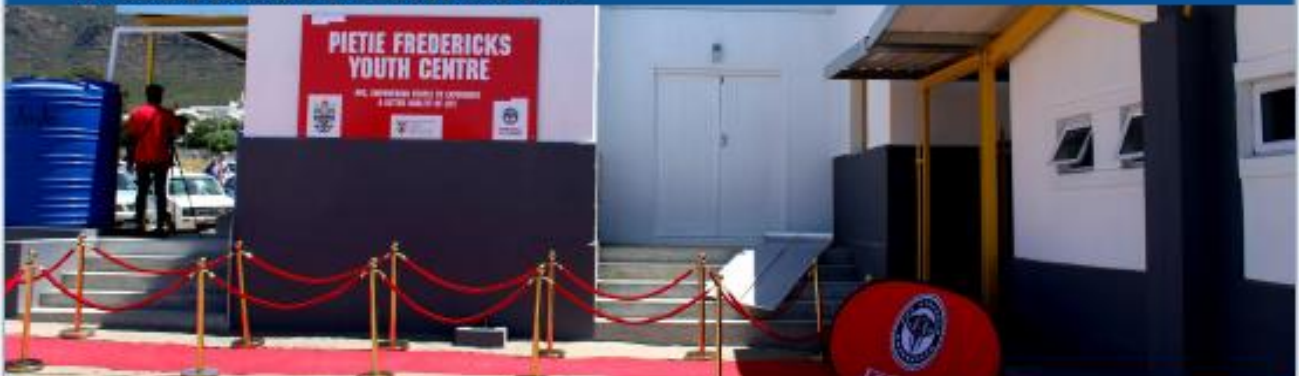
The long-awaited Pietie Fredericks Youth Centre in Piketberg has officially been handed over by PPC De Hoek to Bergrivier Municipality on Monday, 31 October 2022. The first phase has already been completed, however, the second phase is still in progress. This centre will focus on youth development and youth empowerment.
