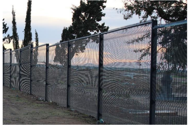
Clearvu fencing at Cemetery No. 2 Piketberg
