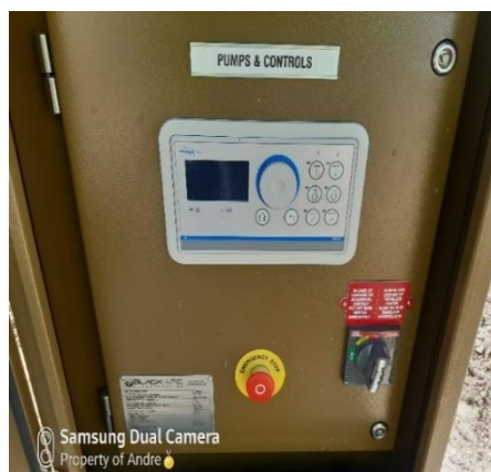
New MCC panels installed at pump stations
