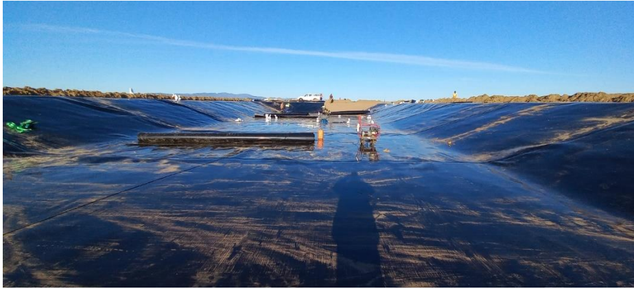
Upgrading of Dwarskersbos Sewerage Works
