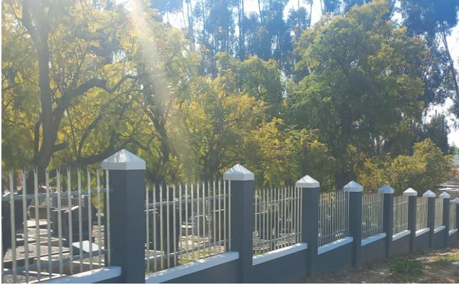
Boundary wall at Old Cemetery Porterville
