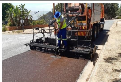
Road being resealed in Piketberg as part of preventative maintenance
