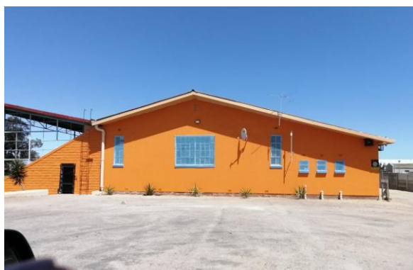
Maintenance at Facilities: Smit Park Sportsgrounds in Velddrif
