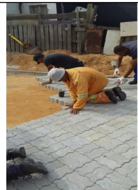
Brick paved construction
