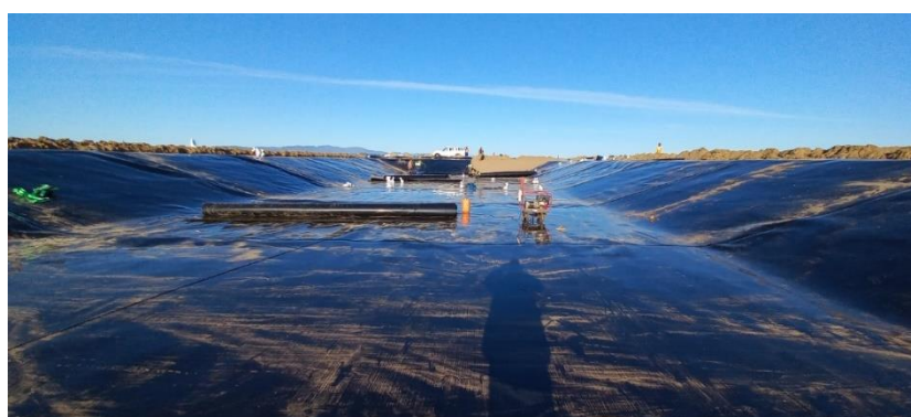
Upgrading of Dwarskersbos Sewerage Works
