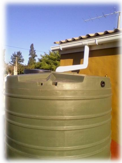
The gutter, downpipe and the tank on the platform in Redelinghuys
