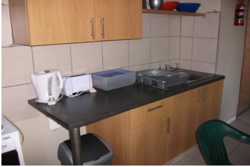
New build-in kitchen cupboards at Rondavels (DKB)
