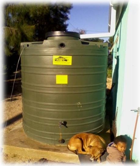
The gutter, downpipe and the tank on the platform in Redelinghuys
