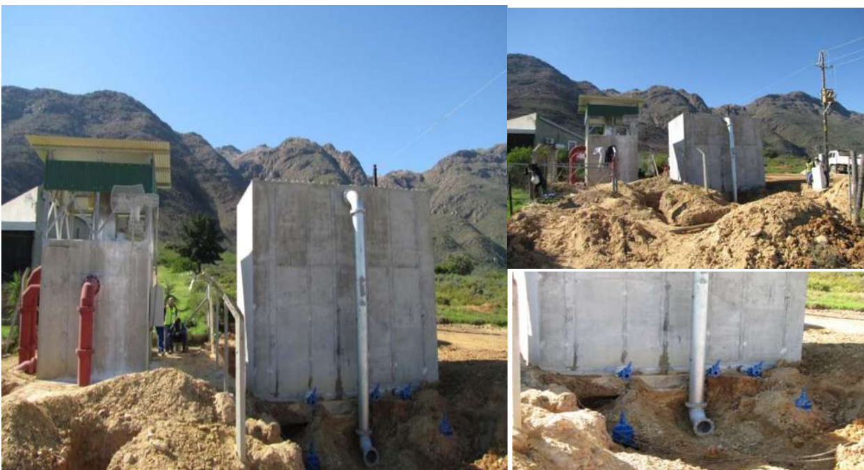
Water Infrastructure Upgrade – Porterville (Photo provided by Rassie Bothma)
