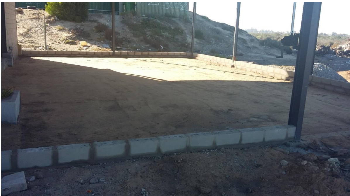
Extension of recycle plant Velddrif
