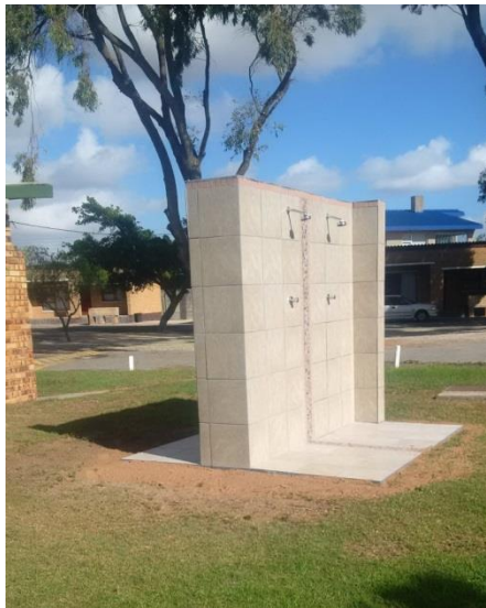
New outside shower at Dwarskersbos beach resort
